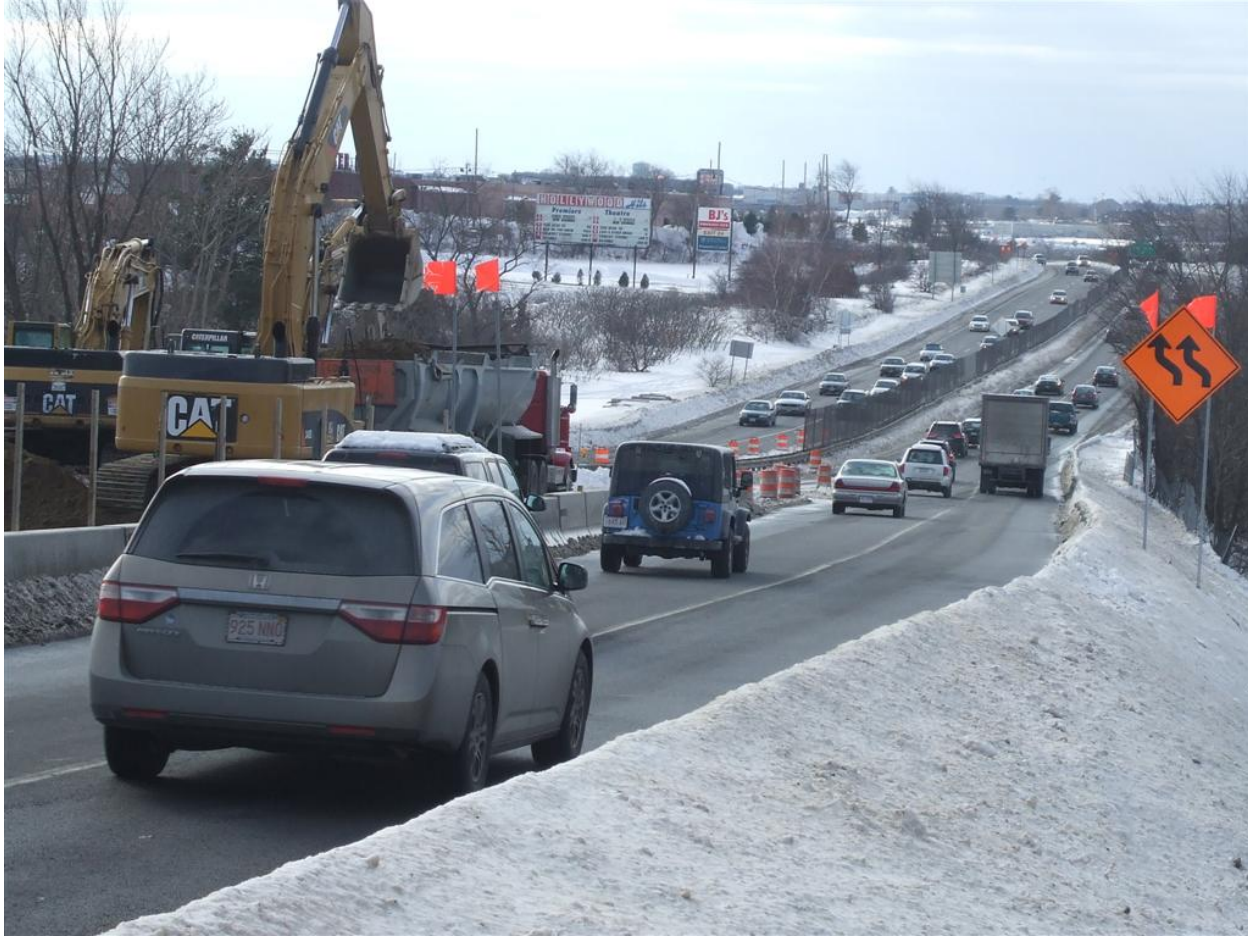
Temporary Route 128 travel lanes constructed as part of the revisions to the traffic management plan to allow the bridge replacement to proceed on an expedited schedule. Photo depicts conditions on Route 128 Southbound. A similar configuration is in place for Route 128 Northbound.
